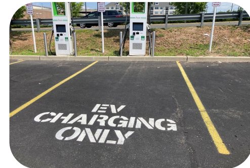
EV Charging Spaces
